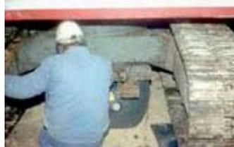
Right on such operations the advantage of air-lift pumps is appreciated when a load can be easily pushed something sideways. With hydraulic tools one would need for this work one whole day, with LAMPE-LIFTERS the work is done within max. 2 hours.
